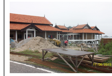
6. Construction of Rest House
