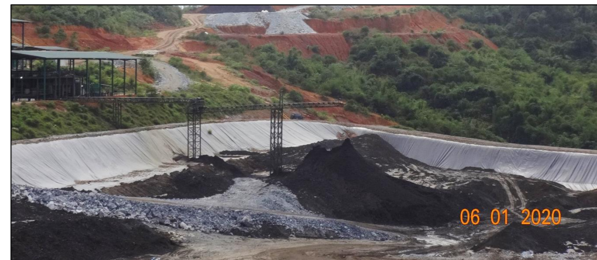
Spent Ore Dump (SOD) underlain with HDPE Geomembrane
