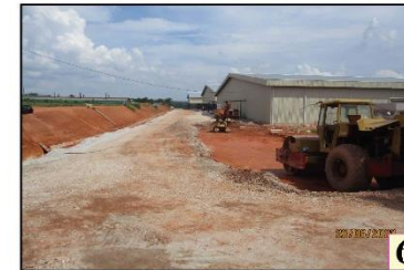
Main entrance of the Proposed Project Site
