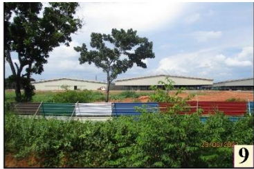
Hoarding along the western boundary of the Project Site
