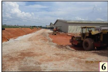
Main entrance of the Proposed Project Site
