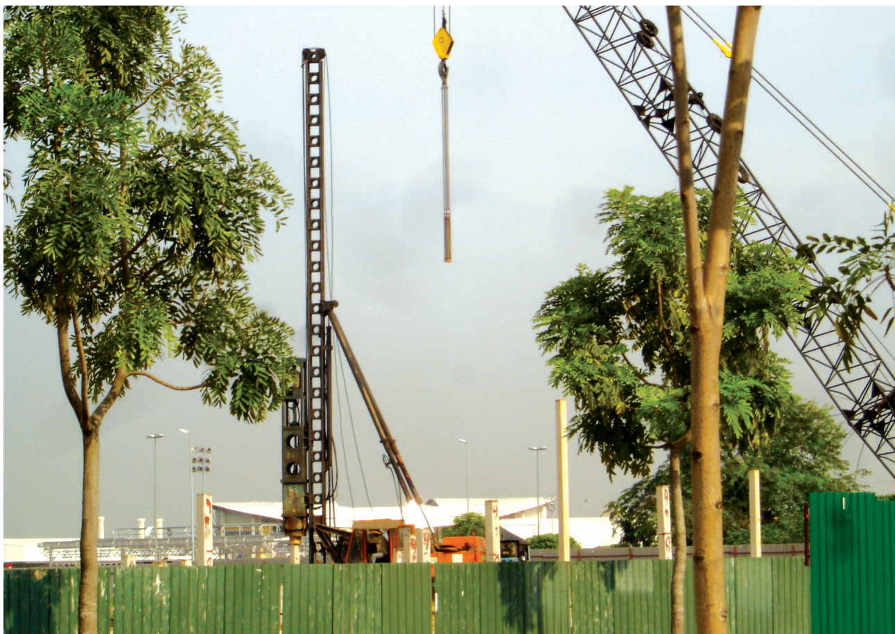
Noise pollution : Hydraulic piling activities (DOE Photo Library)
