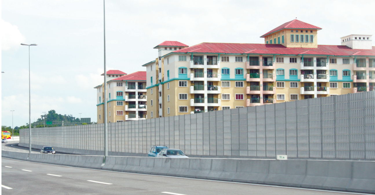
Noise isolating barrier walls installed along the highway (DOE Photo Library)
