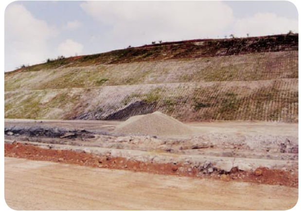
Gambarfoto 4.2 JAS: Menanam Penutup Bumi Sebagai Kaedah Mencegah Hakisan Tanah di Lereng Bukit Photo 4.2 DOE: Cover Crop as a Soil Erosion Prevention Technique
