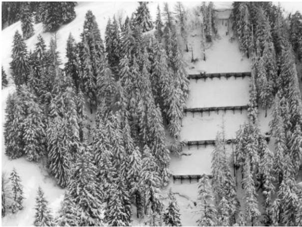
Figure 8 Avalanche starting zone in a gap within the forest protected with wooden defense structures in the Taminatal, Switzerland. The design life of such temporary wooden constructions is at least 50 years and allows time for young trees to become well established.
