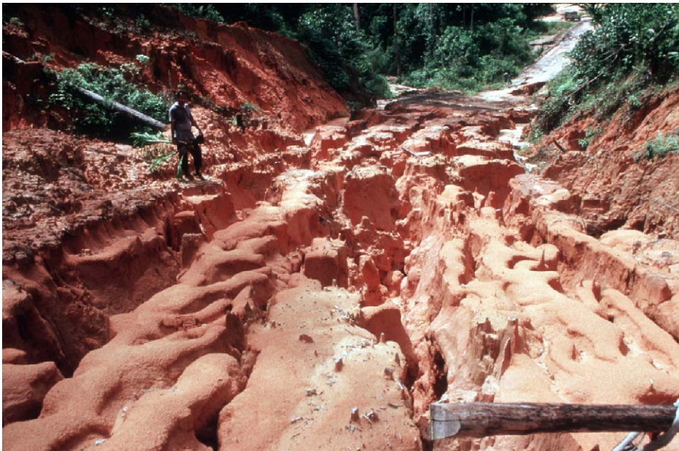
Figure 1 Rills are regarded as the primary detachment agent in water erosion processes. Rill development can be exacerbated in forestry operations due to compaction and vehicular traffic on road and track surfaces. Photograph courtesy of estate of TC Whitmore.
