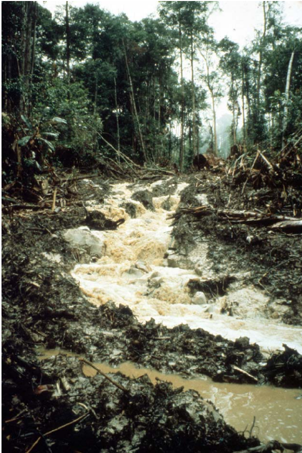
Figure 3 Overland flow develops rapidly on compacted road surfaces that have infiltration rates in some environments as low as 1 \text{ mm h}^{-1} . Photograph courtesy of A Malmer.
