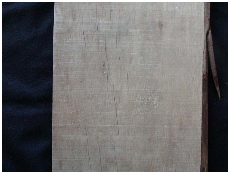
Figure 3 Surface checks can occur if the surface of the board shrinks too much or too quickly compared to the center. This can happen early in lumber drying and the checks close part way through the drying cycle. They are still considered a defect after they close.
