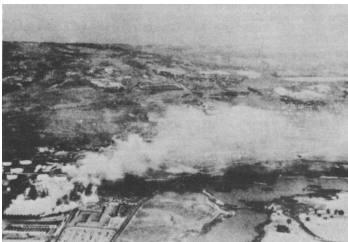
Fig. 10.12. Uncontrolled petroleum refinery.
