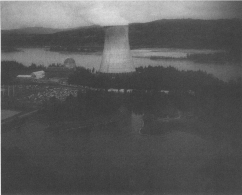
Fig. 31.3. Trojan nuclear power plant. Source: Portland General Electric Company.
