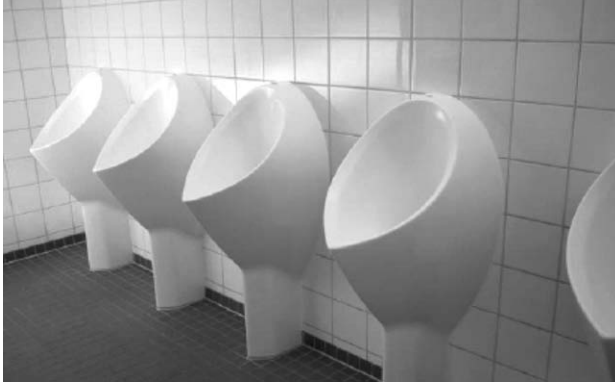
Figure 10.8 A bank of Uridan (fixed cartridge type) waterless urinals Courtesy of Watersave Australia Pty Ltd.
