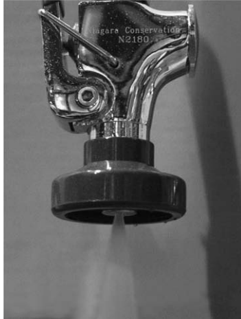
Figure 10.11 A photo of a low flow pre-rinse spray valve in action
