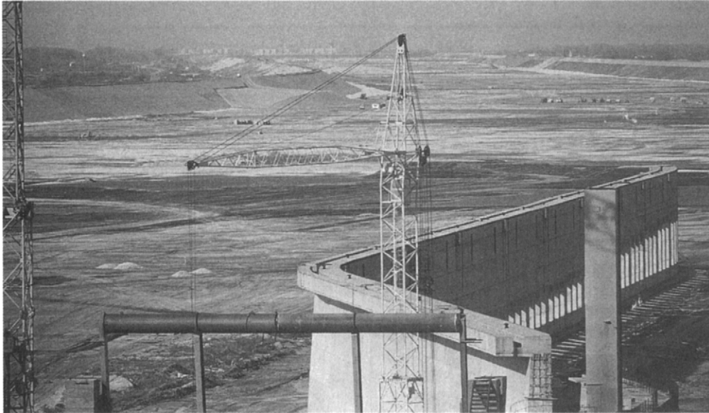
Plate 3.2 Construction work on the Gabčíkovo-Nagymaros dam. Photo: Jacques Langevin/ABC Press
