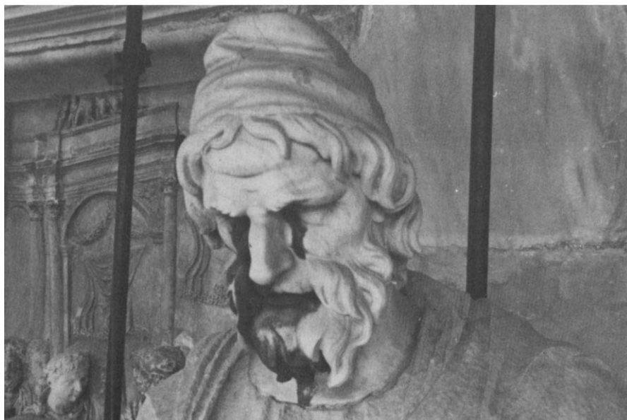
Fig. 3. Examples of white and black areas due respectively to the run-off on the surface (white areas) and deposit of carbonaceous particles and sulphation of the underlying surface in the zones wetted by airborne droplets and percolation, but prevented from run-off (black areas). Their shape is determined by the geometry of the monument. (a) Capital of the Ducal Palace in Venice. (b) Statue on the Constantino's Arch in Rome.
