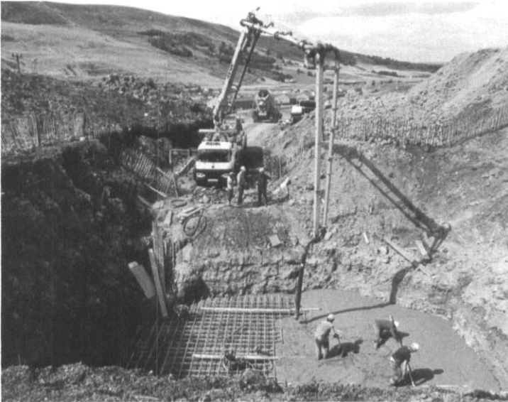
Photograph 3.5: Capping of a mineshaft (source: Richards, Moorehead and Laing Ltd)
