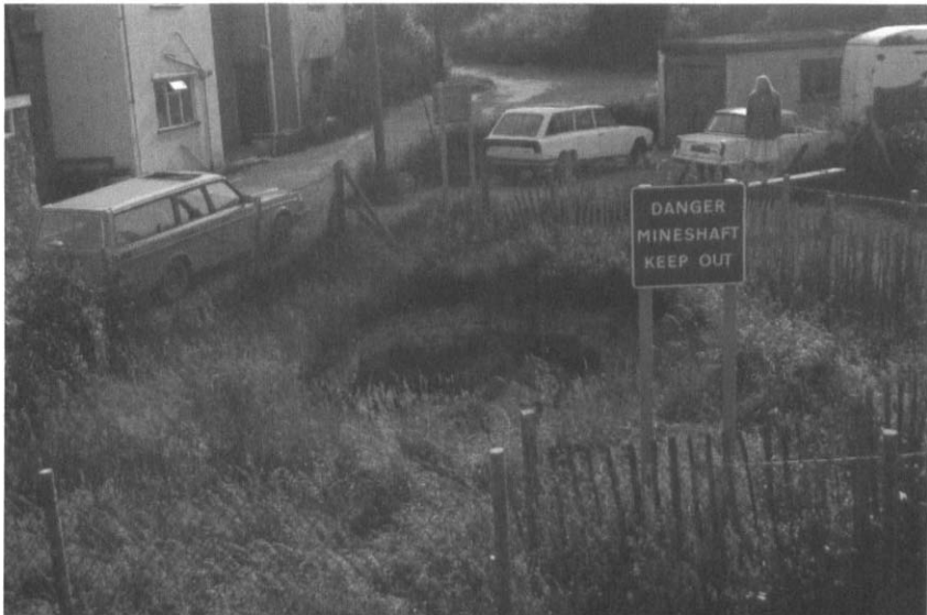
Photograph 3.3: Collapsed mineshaft (source: Richards, Moorehead and Laing Ltd)
