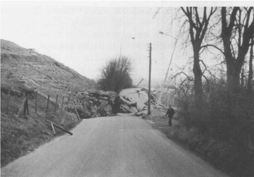
Photograph 6.1: Example of a rotational slip failure (source: I.G. Brown)
