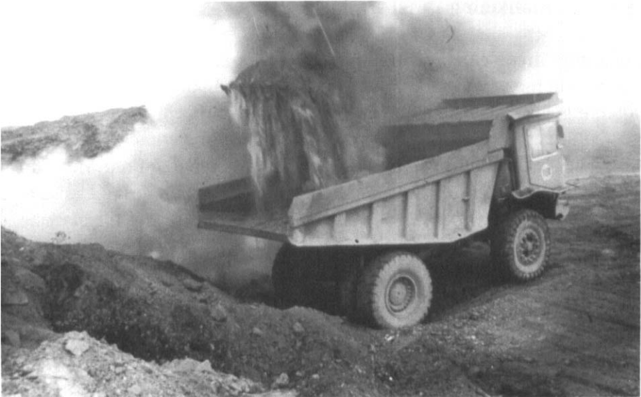
Photograph 7.1: Treatment of a spoil heap fire by excavation (source: Richards, Moorehead and Laing Ltd)
