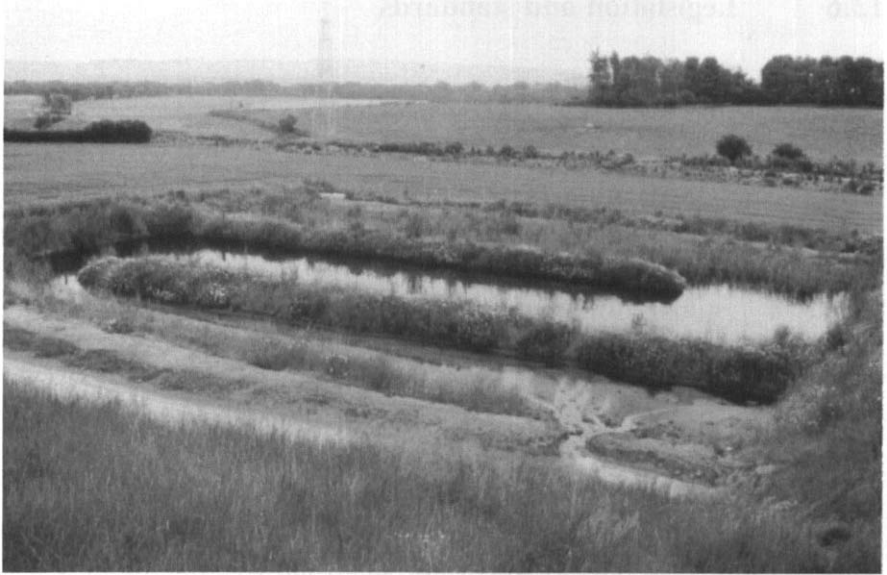
Photograph 12.1: The wetland treatment area at Gilmerton Bing, Lothian, UK. Water draining the colliery spoil enters the lagoon in the foreground from the anoxic limestone drains. Phragmites australis can be seen in the third lagoon of the system (source: Landscape Development).
