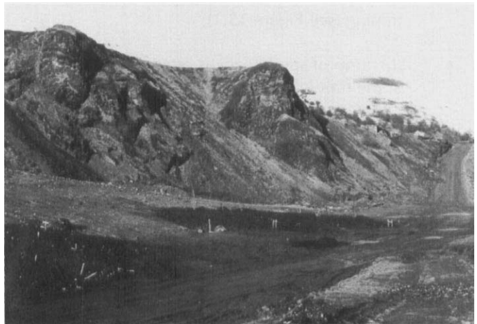
Photograph 13.6: These 'bluffs' formed of steel slag tipped in a molten state, were retained and utilised as a dramatic feature in the 1992 Garden Festival, Wales, UK (source: Richards, Moorehead and Laing Ltd)
