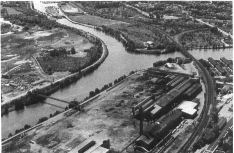
Photograph 13.4: Steelworks typically require a large area of level or terraced land, because of their size, and a good supply of water. This steelworks is already partially demolished (source: Richards, Moorehead and Laing Ltd)
