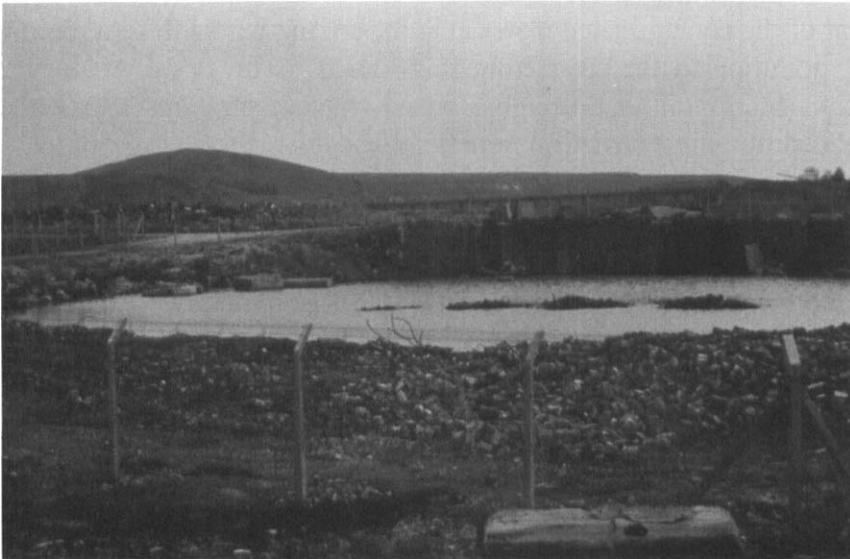
Photograph 17.2: Flooded gas holder base at Orgreave coke works, with Orgreave tip in the background (source: Richards, Moorehead and Laing Ltd)
