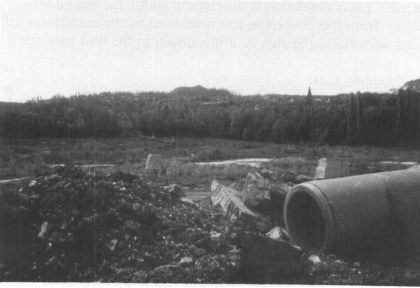
Photograph 17.12: The Aciérie LD site part way through reclamation. The drainage system is being installed (source: Richards, Moorehead and Laing Ltd)
