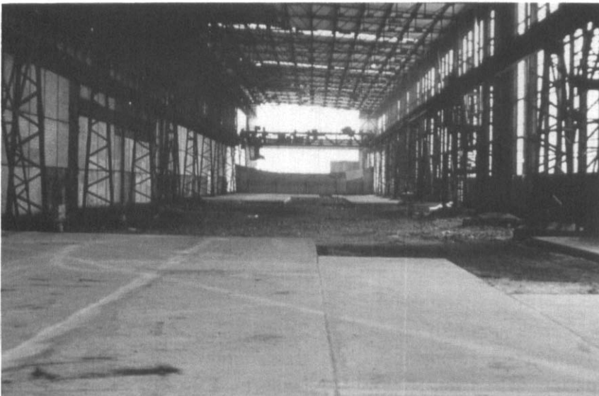
Photograph 17.13: Former steel mill undergoing refurbishment (source: Richards, Moorehead and Laing Ltd)
