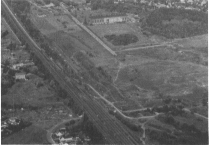
Photograph 17.15: Aerial view of Sachsen mine, Hamm. The large building is the machine hall, the only building on the site which has not been demolished (source: AHU)
