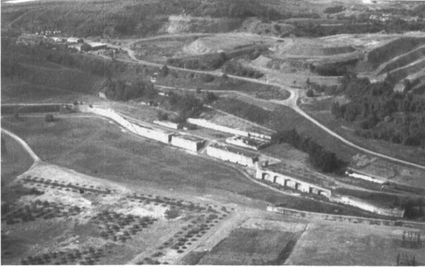
Photograph 17.5: Micheville. Aerial view of the steelworks site following reclamation and initial landscape works (source: EPML)
