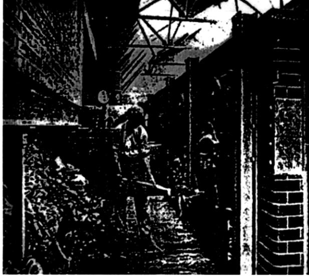
Figure 1.2 Manual Feeding of a Unit at the Glasgow Incinerator Facility
