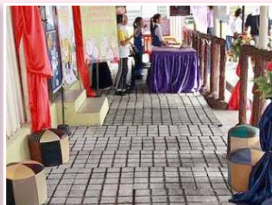
These floor mats, made from rubber and rice husk, were salvaged from another building and reused in the school. Source: The StarOnline.
