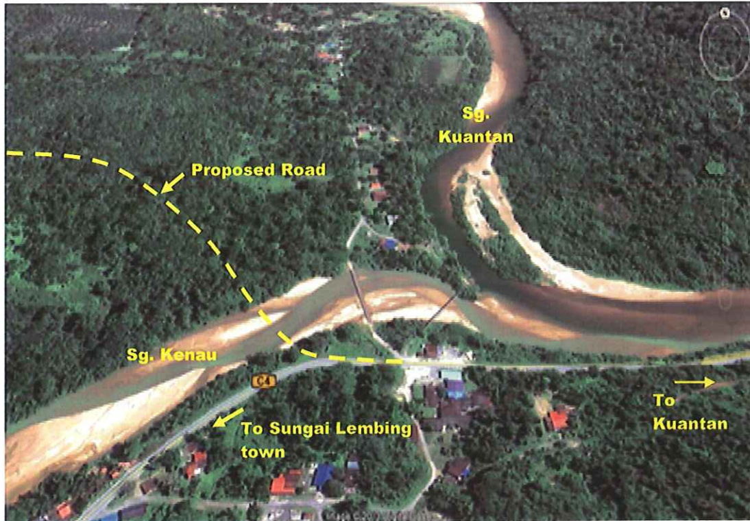
Figure 4.7.1: Aerial view showing road at the eastern side at Sungai Lembing where the proposed road starts
