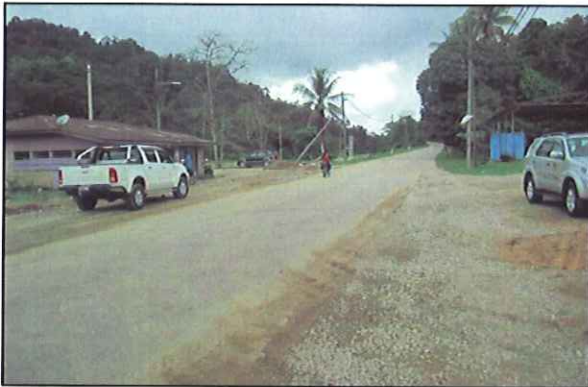
Plate 4.8.1: State road C4 near Kuala Kenau, Sungai Lembing.
