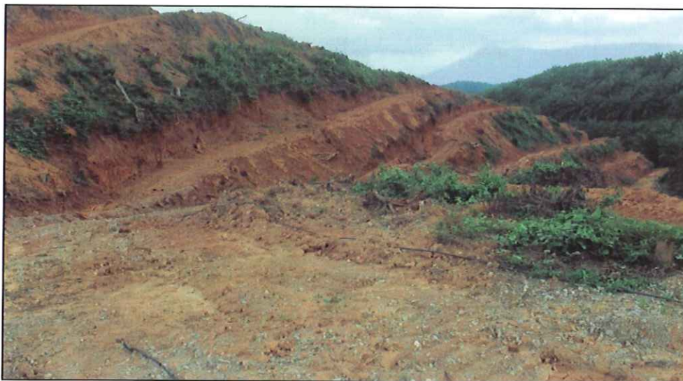
Plate 4.6.4: Cut hill slope exposing very thick weathered granite soil observed at LP01.
