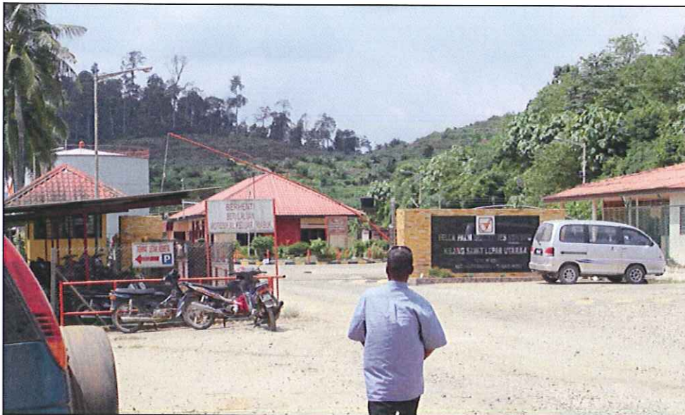
Plate 5.9.1: Kilang Sawit Lepar Utara 4.
