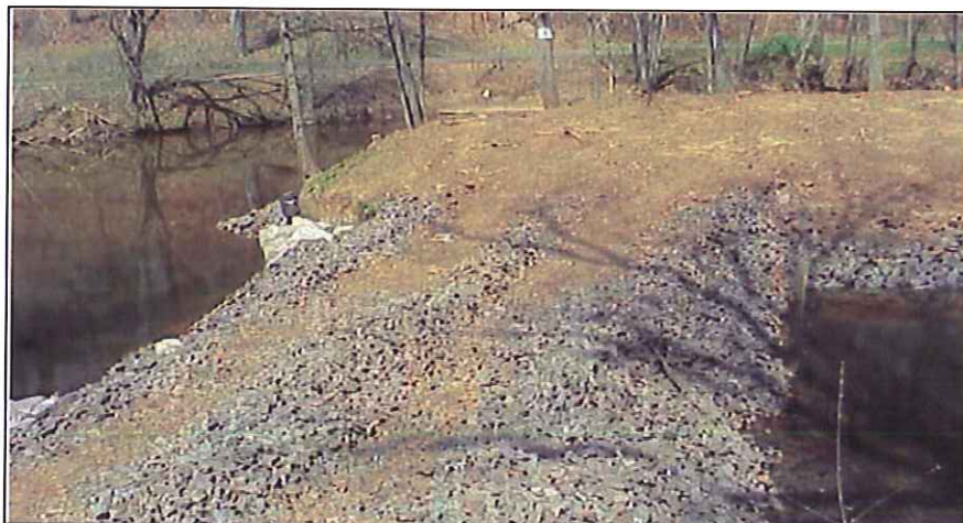
Plate 6.4.2: Temporary Waterway Crossing
