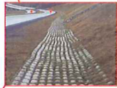
PERMANENT SWALE WITH BED PROTECTION
