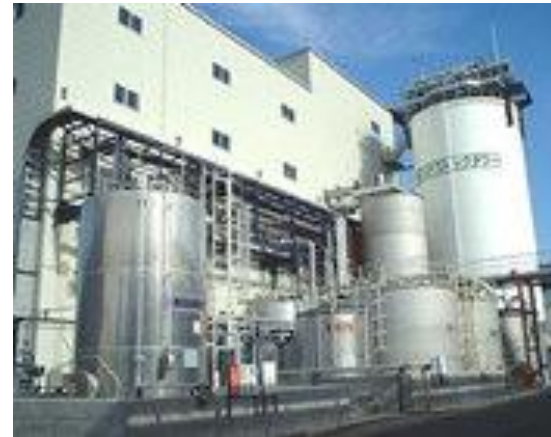
Stock tower of recycled pulp
