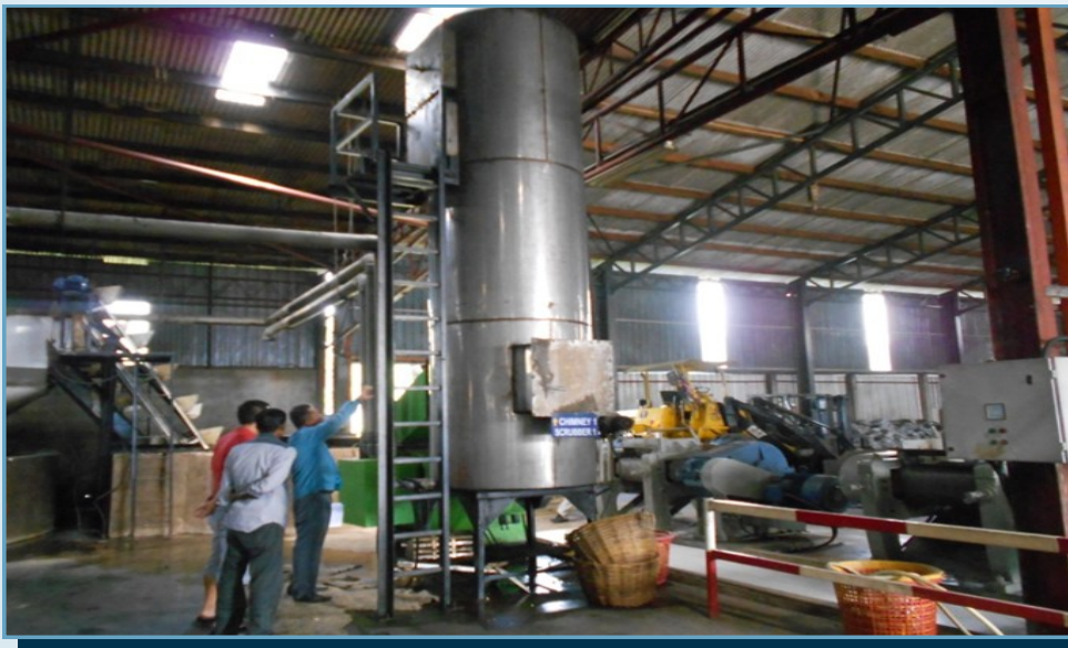
Alat Kawalan Pencemaran Udara Scrubber Kilang Memproses Getah
