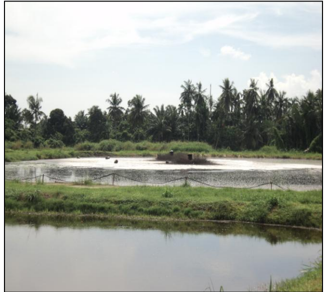
Gambarfoto 3.2: Sistem pengolahan efluen (Aeration Pond)
