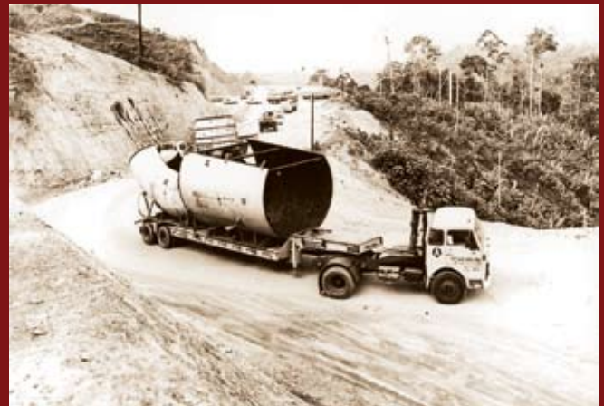
Transporting part of the Penstock from Butterworth to Temengor Power Station for installation. Note the tight escort provided by using heavy armoured vehicles moving in front and behind the transporter.
