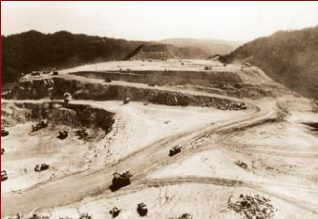
Construction of the Temengor main dam in progress. Work was carried out day and night. The surrounding area of the dam site was guarded by a battalion of infantry 24 hours a day.
