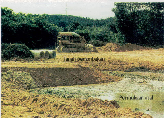
Rajah 2: Proses perataan tanah
