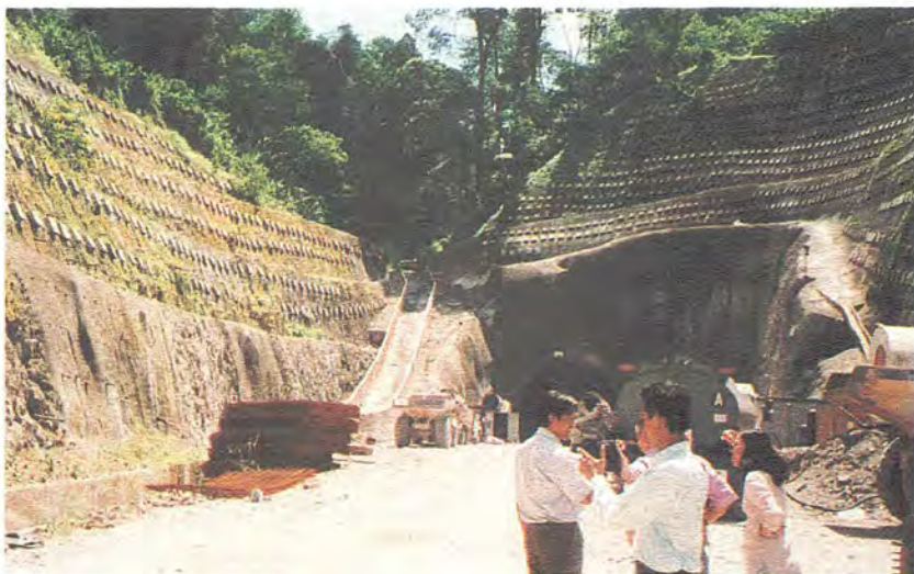
Tunnel Construction at Karak Highway, showing slope stabilization to avoid erosion
