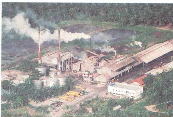
A typical aerial shot during the DOE - Royal Malaysian Police (Air Wing) airborne surveillance
