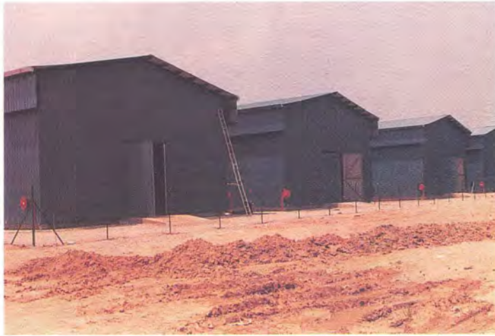
Storage Facilities of Scheduled Waste at Bukit Nanas, Negri Sembilan.
