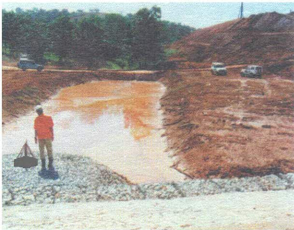
Silt traps constructed for the Putrajaya Federal Development Project.
