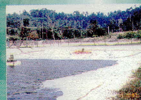
Industrial Wastewater Treatment
