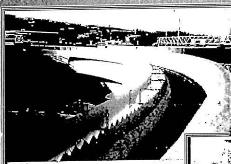
Horizontal Flow Clarifier - circular
