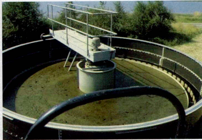
Sedimentation tank
