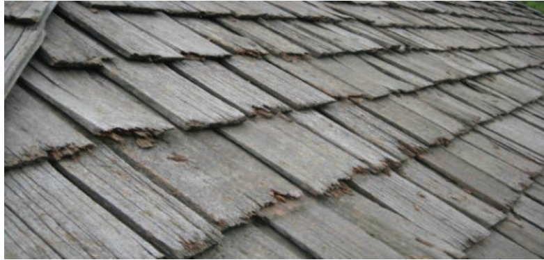
Figure 1.15: Rapid Material Degradation
