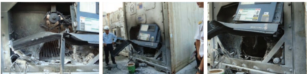
Figure 10.2: Incident caused by misuse of fake refrigerant
