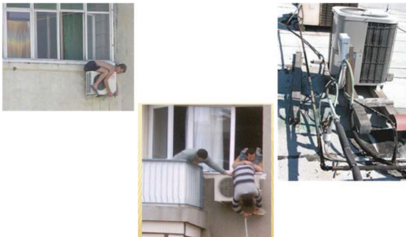
Figure 12.6: Improper installation
