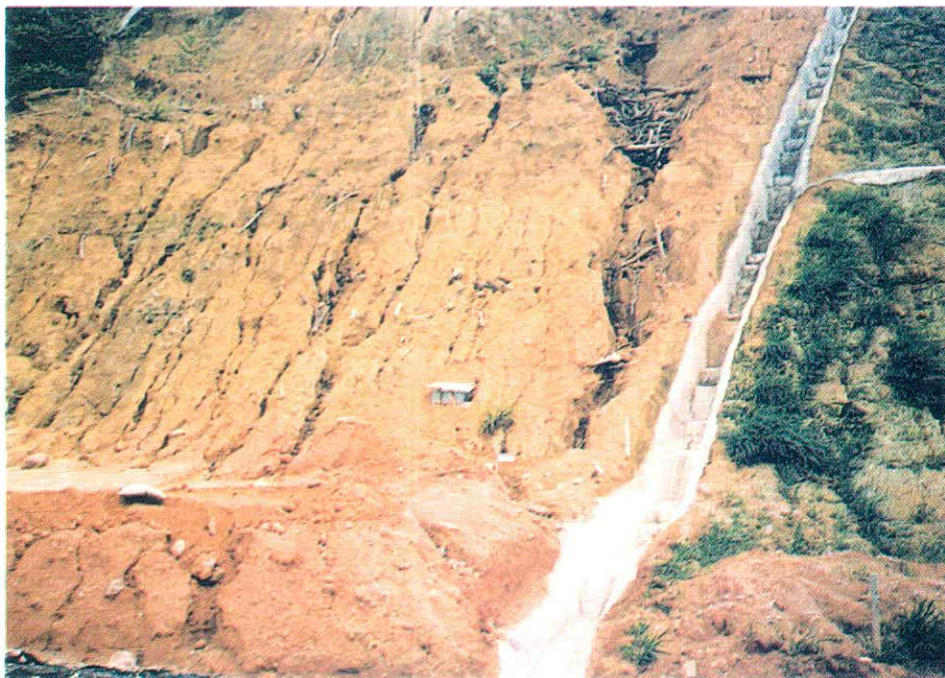
Figure 2.5.3: Rill Erosion
