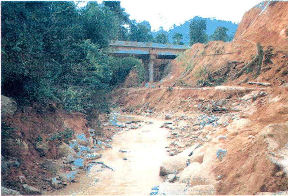
Figure 2.5.5: Riverbank Erosion
