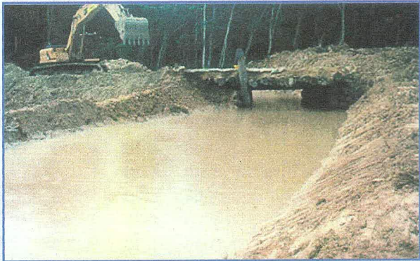
Plate 15: The impact of river deepening on Sg. Tiram in Perak (Turbidity = 250 NTU, SS = 372 mg/l, WQI = 61.2 (Class II))
