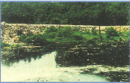
Plate 7: Landfill site as a result of establishment of residential area
