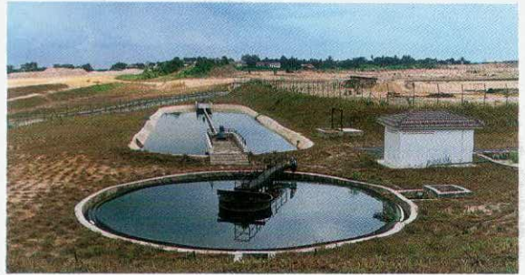
Open ground level design Oxidation Ditch sewage treatment plant for Taman Bukit Mewah, Johor Bahru, Malaysia.
