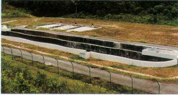
Oxidation Ditch sewage treatment plant for Penjara Sungai Buloh, Selangor, Malaysia.
