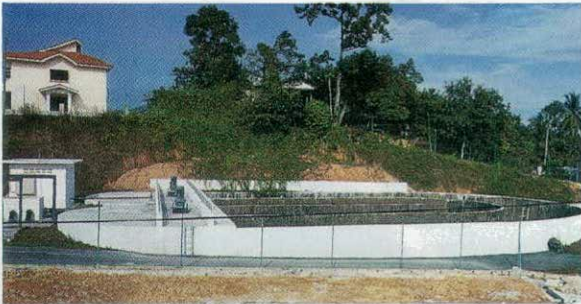
Oxidation Ditch sewage treatment plant for Taman Cheras Utama, Kuala Lumpur, Malaysia.
