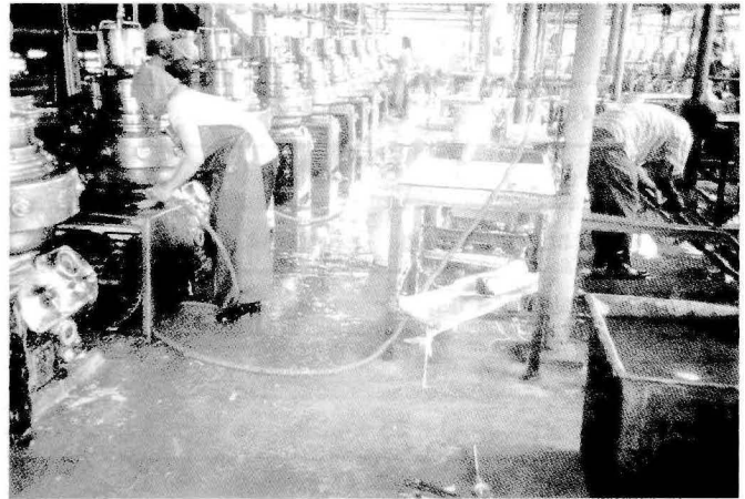
→ Sources of effluent: Washing of equipments
