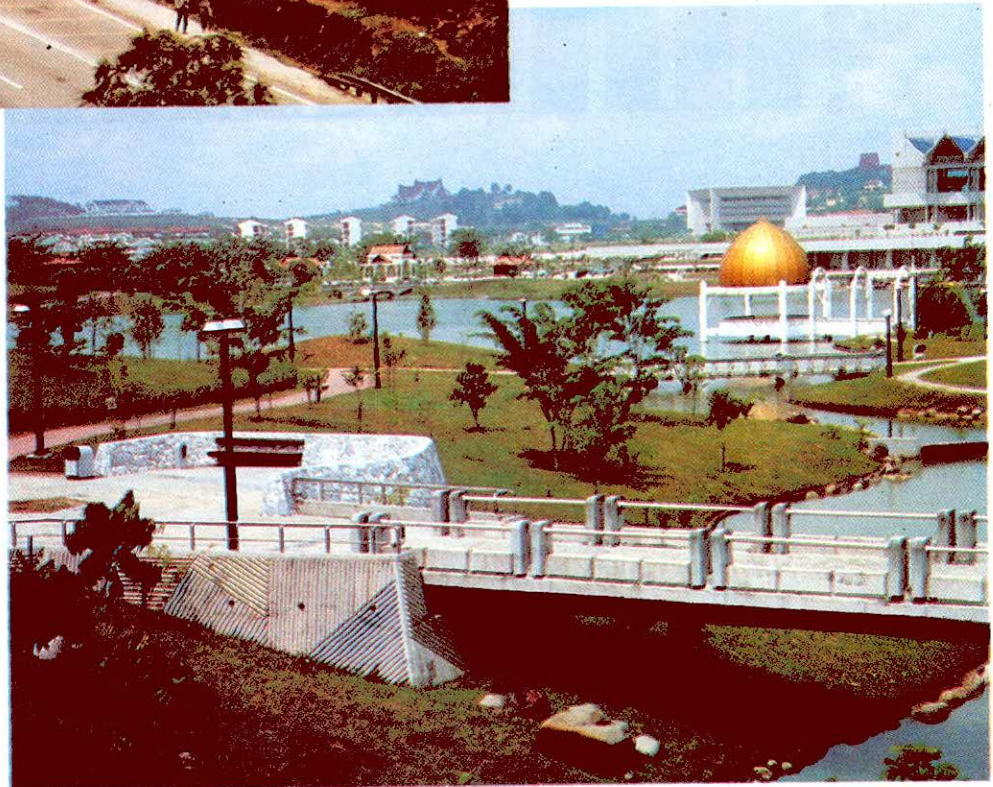
Construction of new townships
