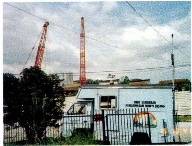
Construction Noise - monitoring by Mobile Unit
