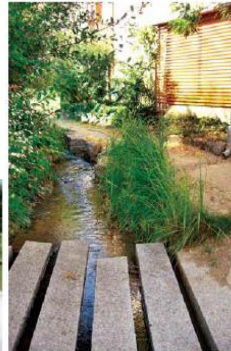
Fig. 4.21 Strips of stones continue the footpath as it crosses the swale. Gaps allow the water to flow in between while the stones are slightly staggered in a playfully sculptural manner (image by Atelier Dreisaitl).
