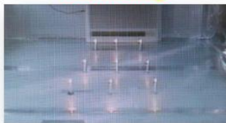
Before R32 leakage
