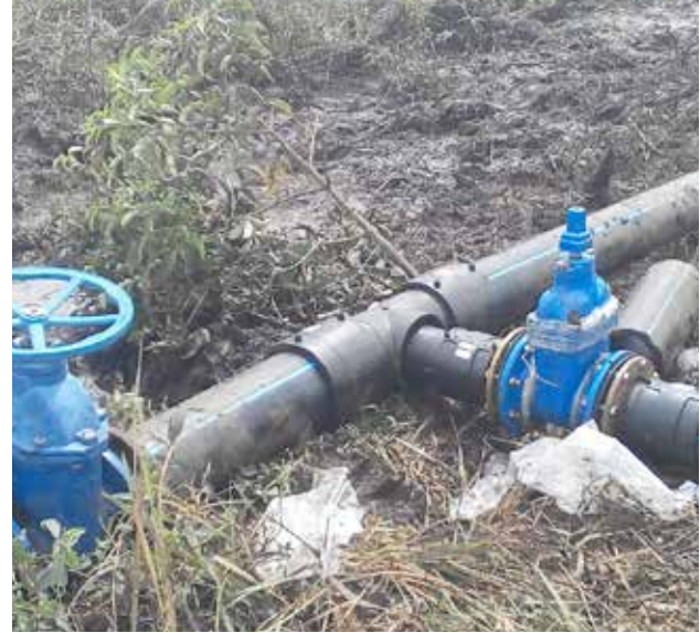
Gambar foto 4.4 : Paip Saluran Air di Hutan Simpan Raja Musa, Kuala Selangor, Selangor bagi meningkatkan paras air gambut Photo 4.3 : Water Piping in Raja Musa Forest Reserve, Kuala Selangor, Selangor to raise peat land water level
