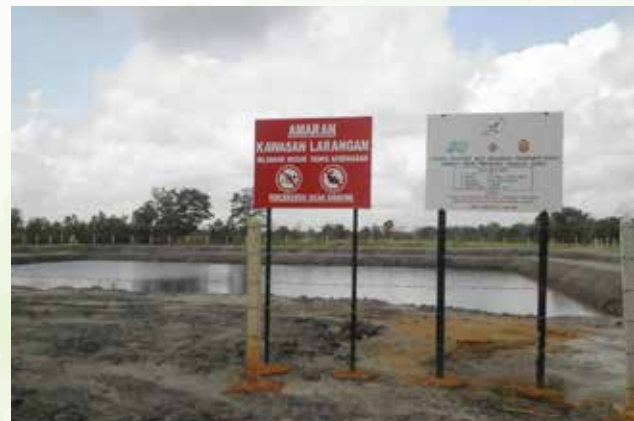
Gambar foto 4.6 : Kolam Takungan di Pekan, Pahang Photo 4.6 : Detention Pond in Pekan, Pahang
