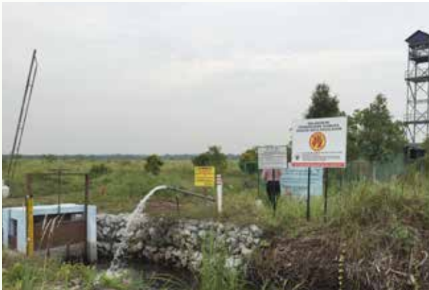
Gambar foto 4.5 : Pengoperasian telaga air tanah, sekatan saluran dan menara tinjau di Kuala Langat, Selangor Photo 4.5 : Operation of tube well, check dam and watch tower in Kuala Langat, Selangor.
