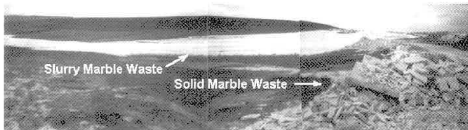
Fig. 9. Overall view of the marble slurry waste storage field at Susuz Boğazi.
