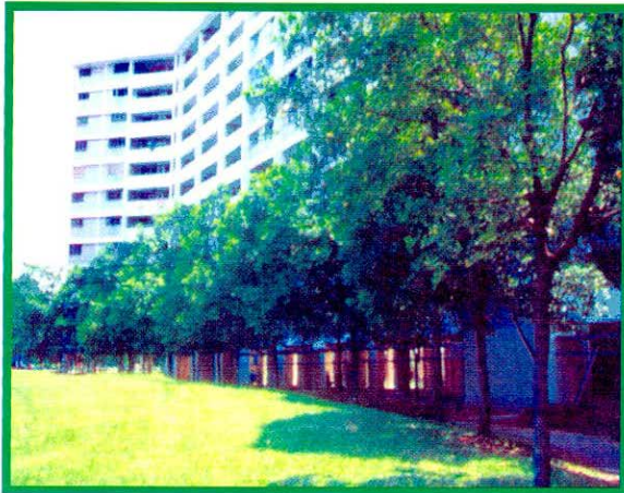
Ten years later, a buffer belt of mature mangroves has firmly established behind the concrete revetment constructed by DID at Sg. Besar.
