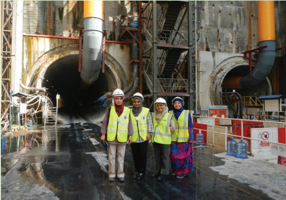
Gambar3(b): Pembinaan Mass Rapid Transit Tunnel
